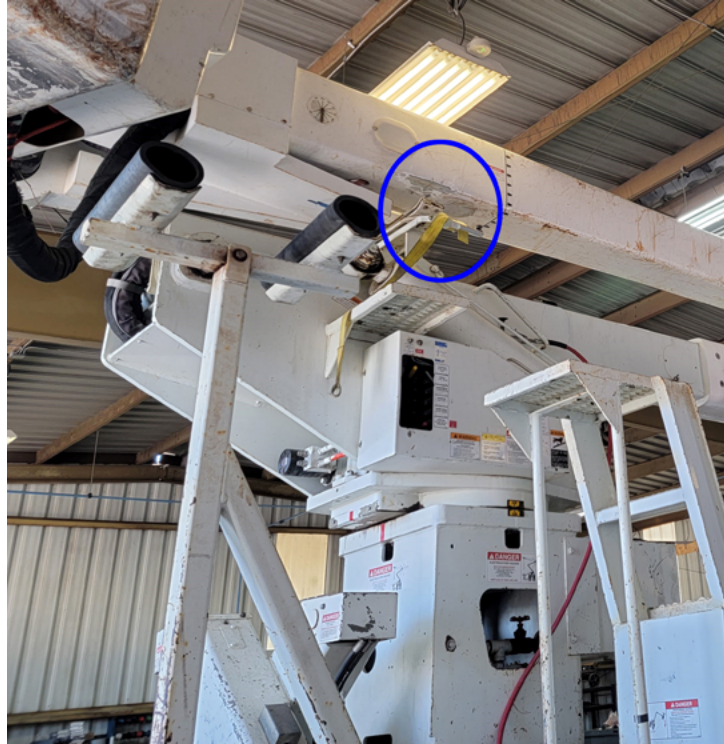
FIGURE 5 - Location of damage showing the boom for perspective
